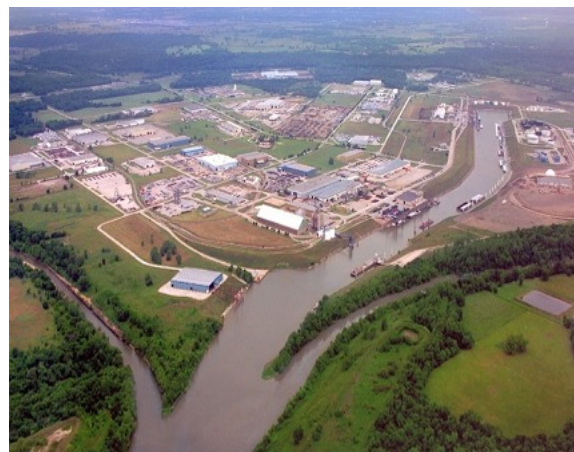
Port of Catoosa on the McClellan-Kerr Navigation System
