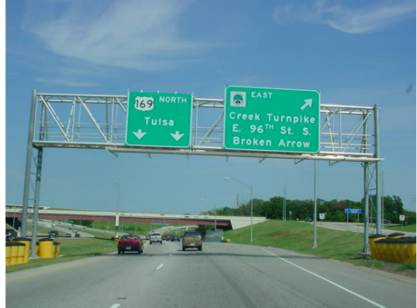
Mingo Valley Expressway (US Hwy 169) at Creek Turnpike interchange
