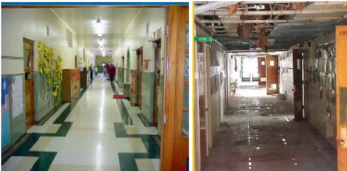
Before and after photos of hallways in Wichita Kansas schools damaged by a tornado
