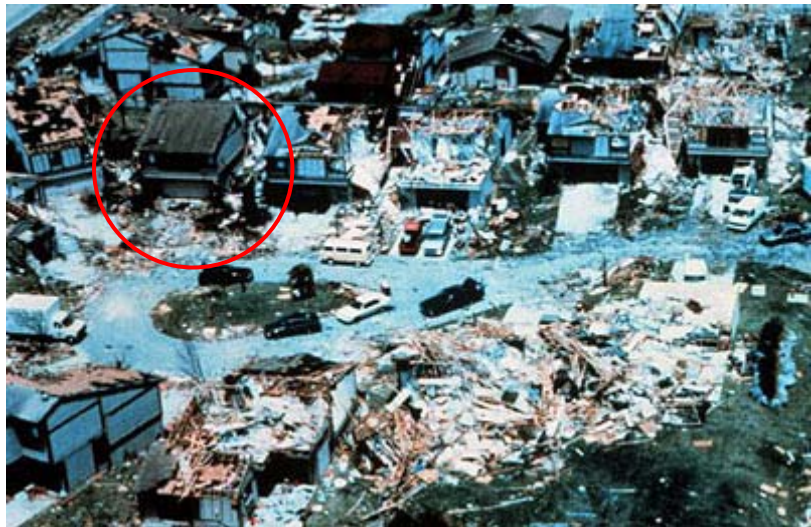
Illustrating the dangers of unreinforced garage doors, in all but the house at upper left, these doors have been breached, leading to substantial roof damage – in some cases, completely removing a second floor. But in the home with an intact garage door, the roof is almost entirely undamaged.
