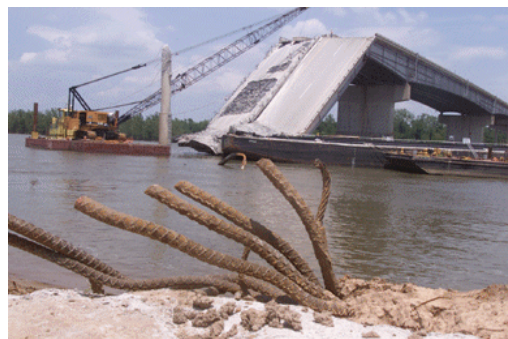
I-40 Bridge collapse at Webbers Falls on the McClellan-Kerr Navigation System of the Arkansas River
