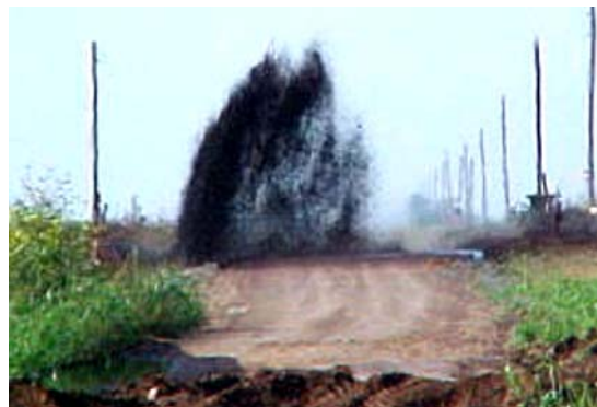
Pipeline break in Jackson County
