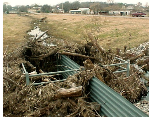
Drainageways should be inspected regularly for blockage from debris
