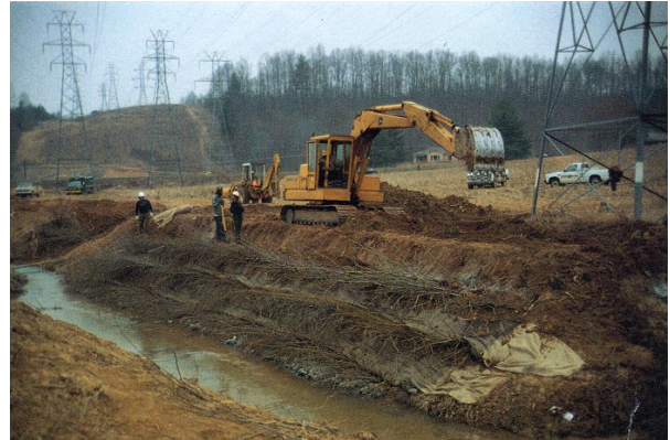
Retrofitting streambanks with willow cuttings and geotextiles can be more cost effective than riprap or concrete-lined floodways.
