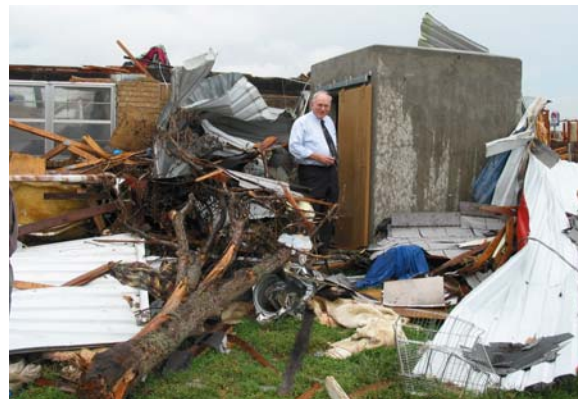
Dr. Ernst Kiesling, Civil Engineering Professor at Texas Tech University, inspects a safe room in the aftermath of the May 8, 2003 tornadoes in Moore, Oklahoma.
