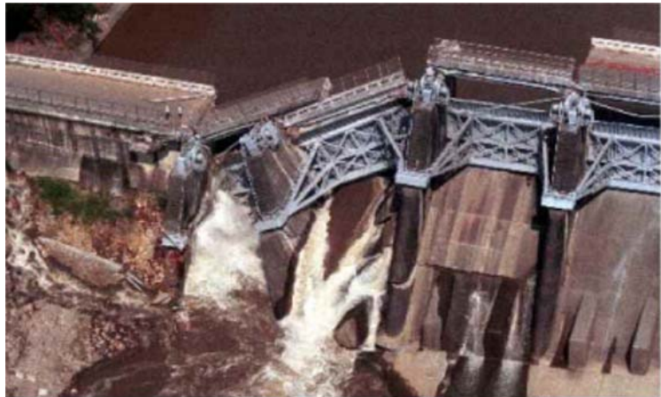
The overtopping or forced release of a dam due to heavy rain or abnormal river flows is a threat to downstream properties.
