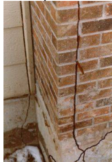
Cracks in a chimney caused by soil expansion
