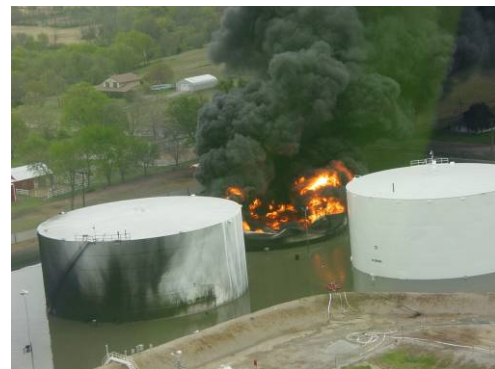
The ConocoPhillips tank fire forced the evacuation of over 400 people.
