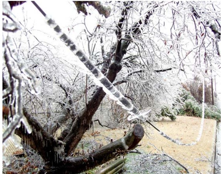
Ice can add up to 500# of weight per line between power poles. (Picture from the Oklahoma 12/2007 ice storms)
